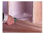
12--A small-diameter roller is used to apply the primer and top coat. The square end of the roller allows it to paint into corners.
