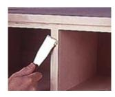
9--Use a putty knife to press drying filler into the nail holes. Slightly mound the filler, and let it harden before sanding.
